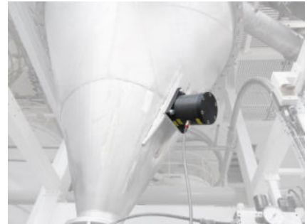
NTS 54/02 for improving material flow
