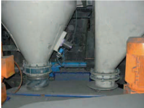
Loosening hard crusts with pneumatic linear vibrators
